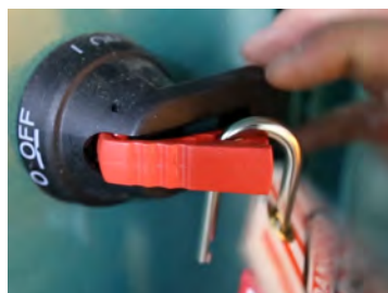
Insert Lock into hole.
